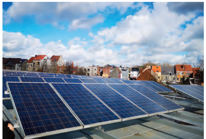
Large roof in Ghent (Belgium) with solar panels installed and operated by Energent. © REScoop.eu
