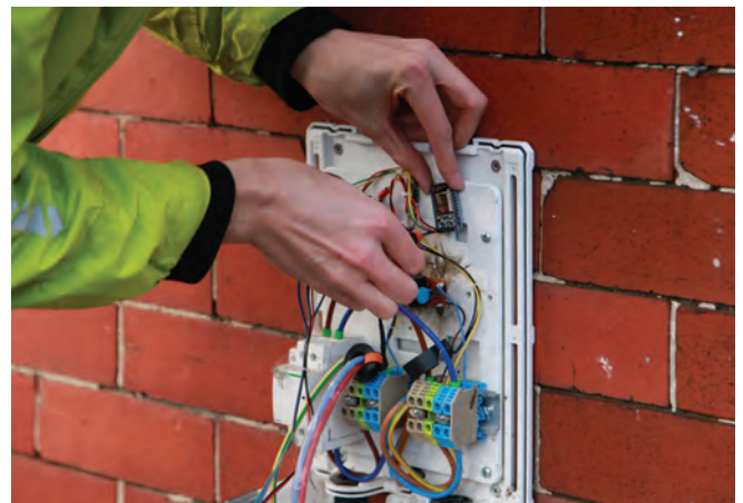
Installation of PowerShaper for automated demand side response. © Carbon Co-op
